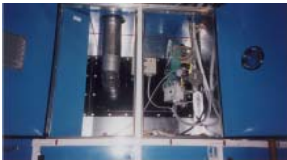
Burner (heat for reactivation) and exhaust
