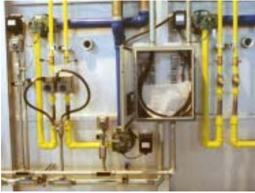
ThermJet Burner Piping Detail
