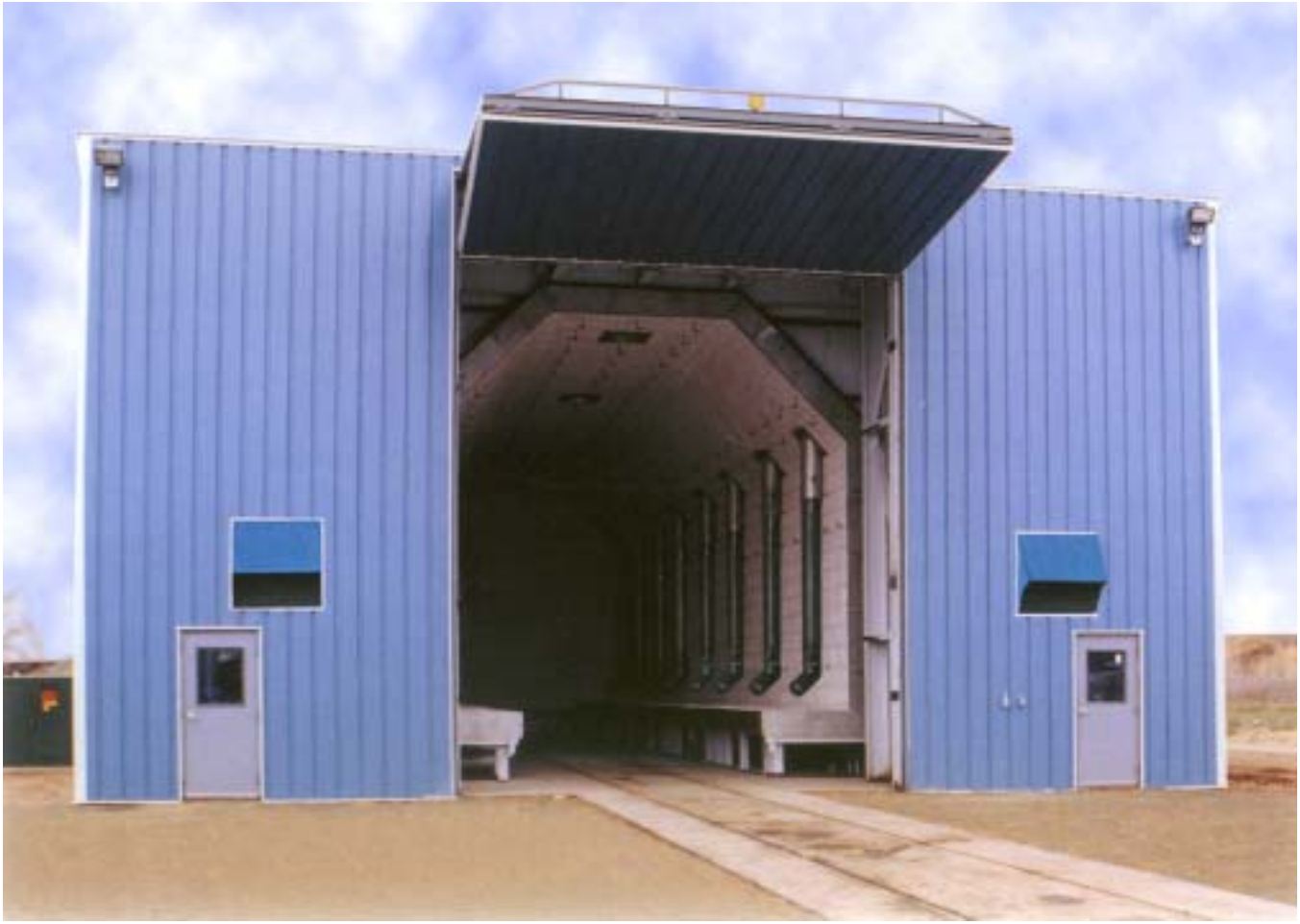
Arrow Tank's Heat Treatment Furnace uses natural gas as its primary fuel and propane as a standby fuel.
